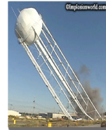
FERNALD WATER TOWER BLASTER - STEVE PETTIGREW DEMOLITION DYNAMICS
