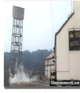
EXTEC TOWER BLASTER - MICK WILLIAMS CONTROLLED DEMO. GROUP, LTD (UK)
